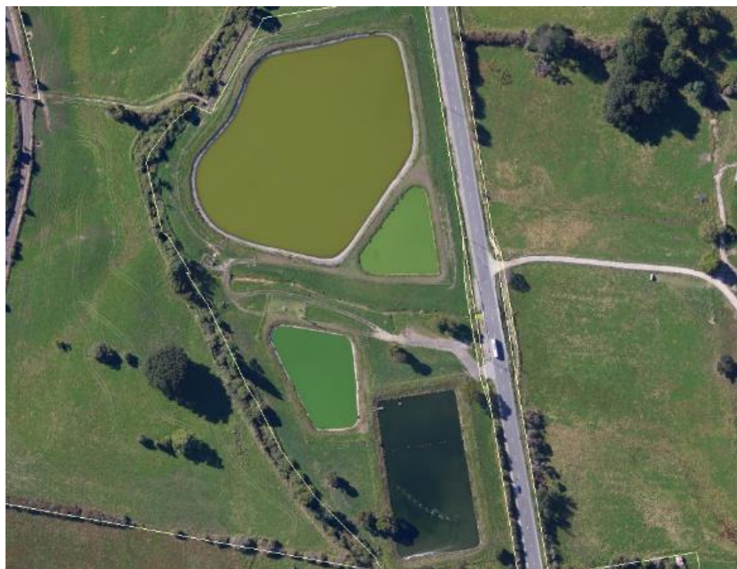
Figure 31--1: Lilydale Sewage Treatment Plant
