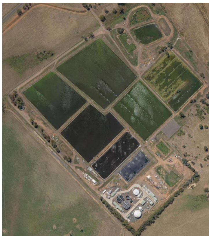
Figure 32-1: Longford Sewage Treatment Plant
