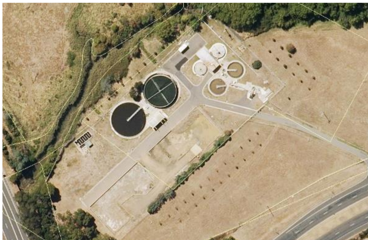
Figure 35-1: Newnham Sewage Treatment Plant
