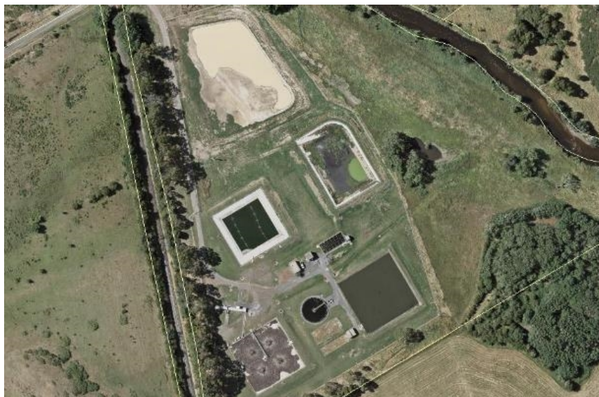
Figure 36-1: Norwood Sewage Treatment Plant
