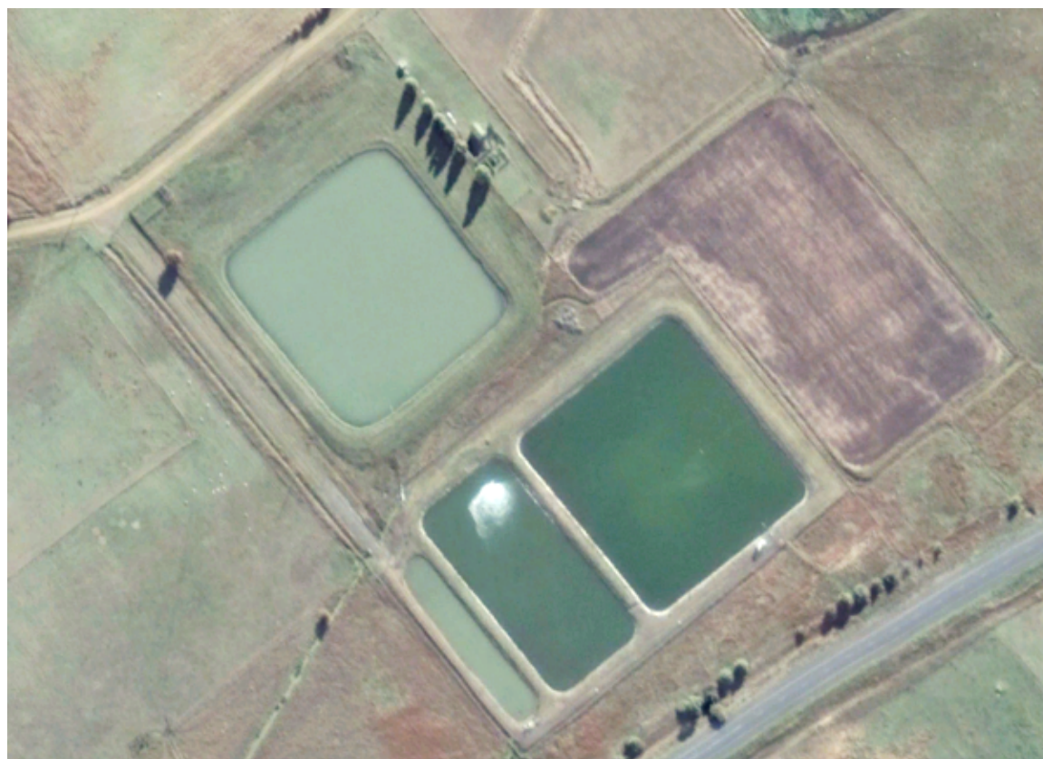
Figure 37-1: Oatlands Sewage Treatment Plant
