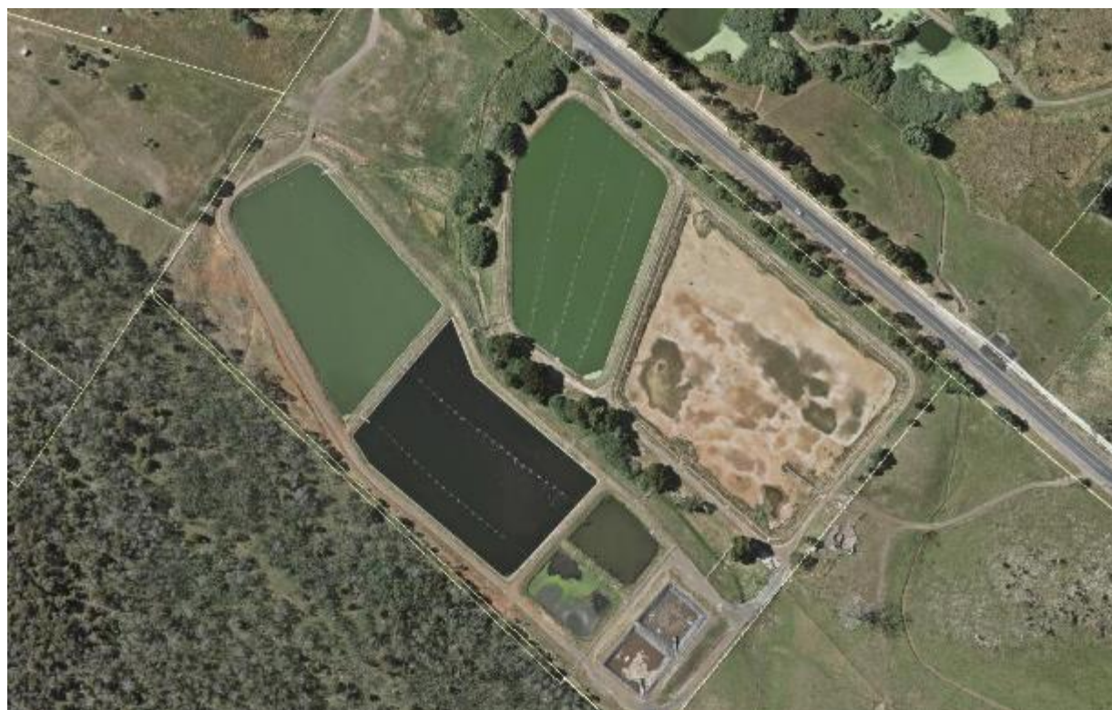
Figure 44-1: Prospect Vale Sewage Treatment Plant
