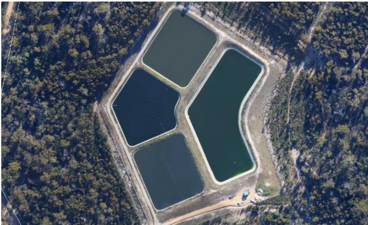
Figure 55-1: Scamander Sewage Treatment Plant
