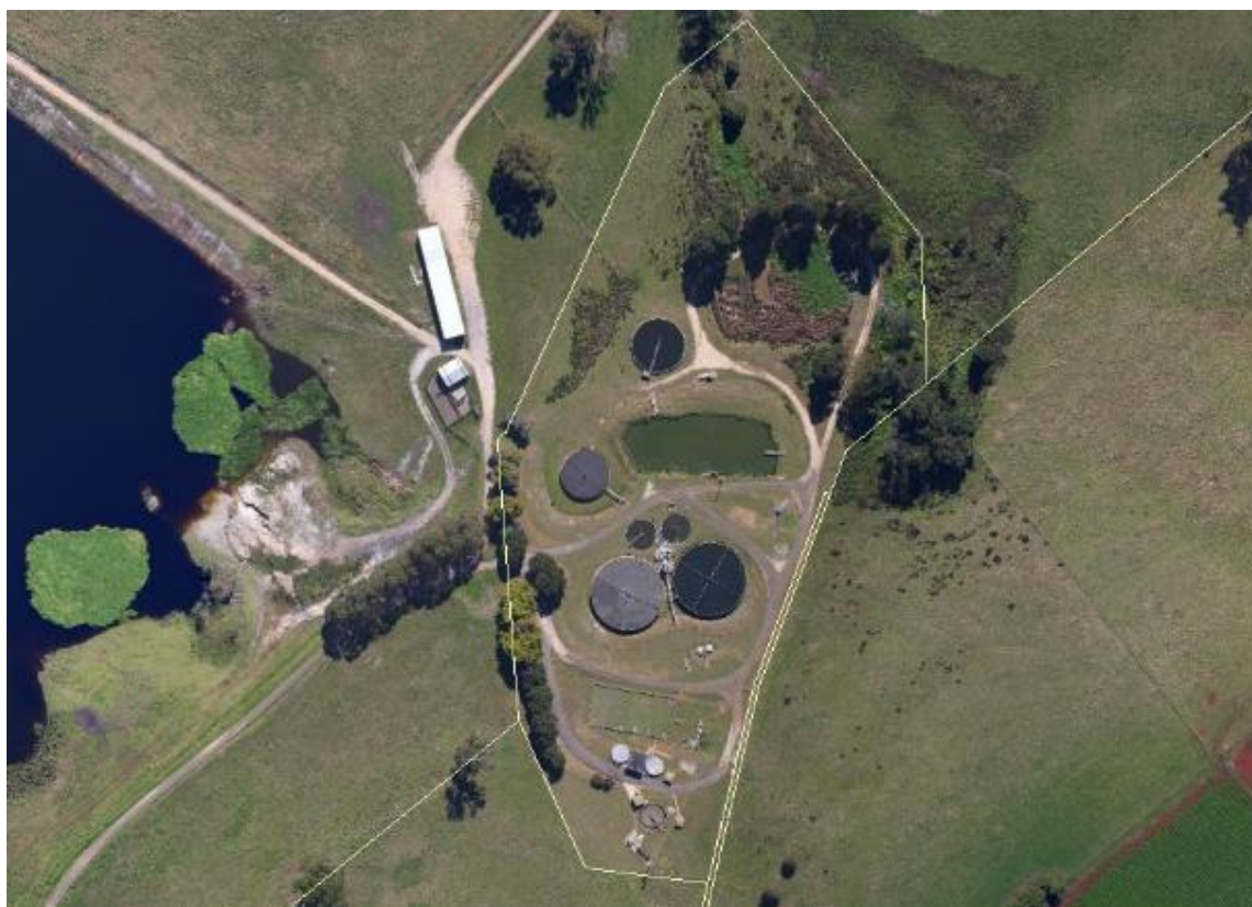
Figure 56-1: Scottsdale Sewage Treatment Plant
