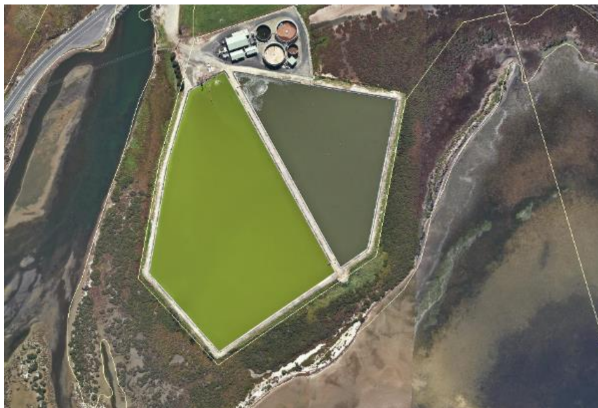
Figure 63-1: St Helens Sewage Treatment Plant
