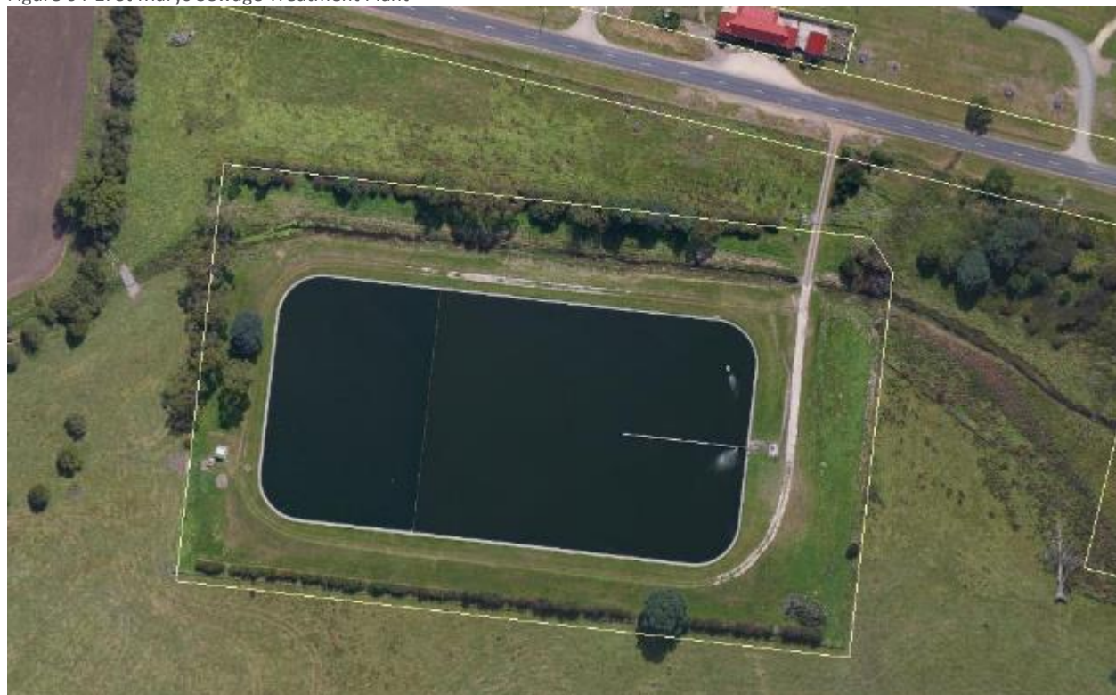
Figure 64-1: St Marys Sewage Treatment Plant
