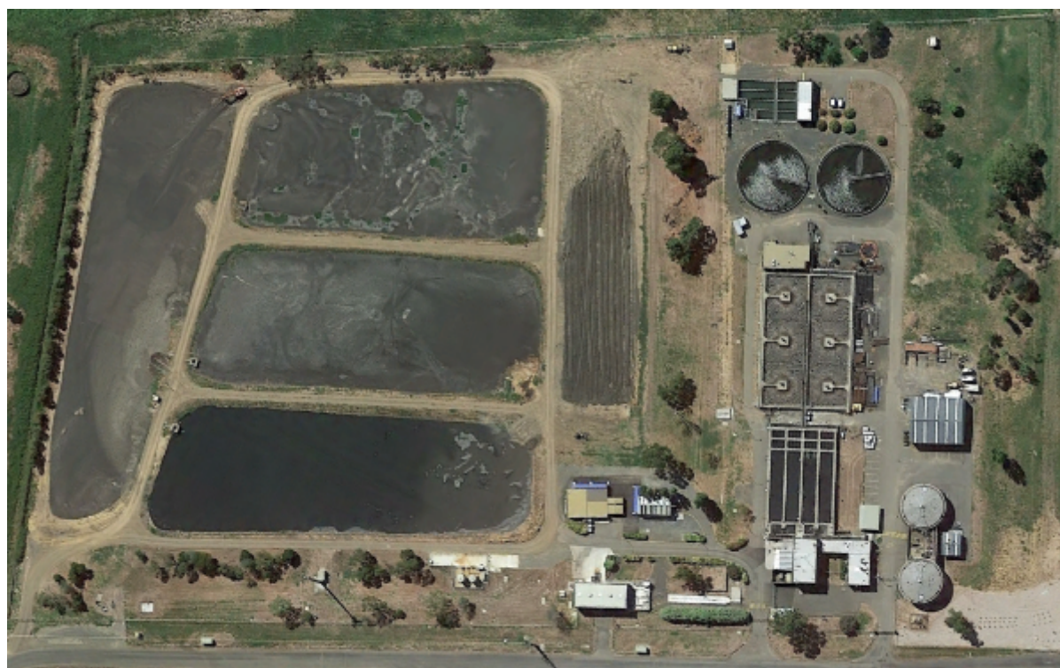
Figure 69-1: Ti Tree Sewage Treatment Plant
