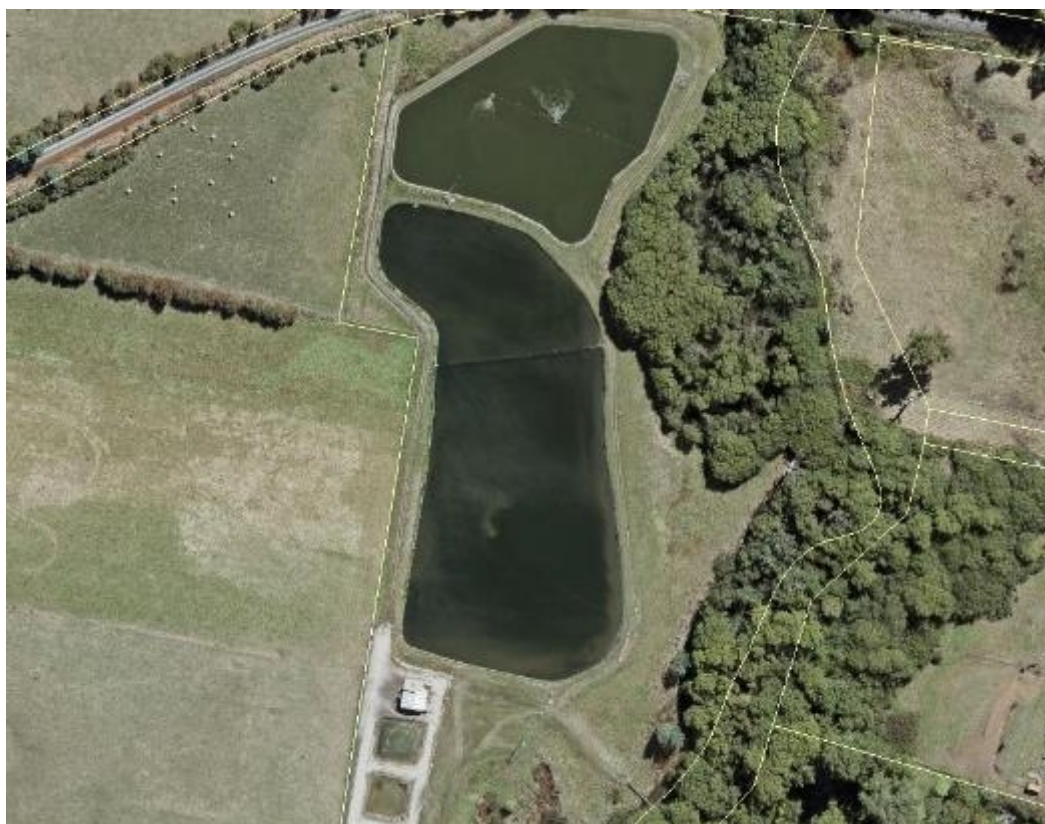
Figure 75-1: Westbury Sewage Treatment Plant
