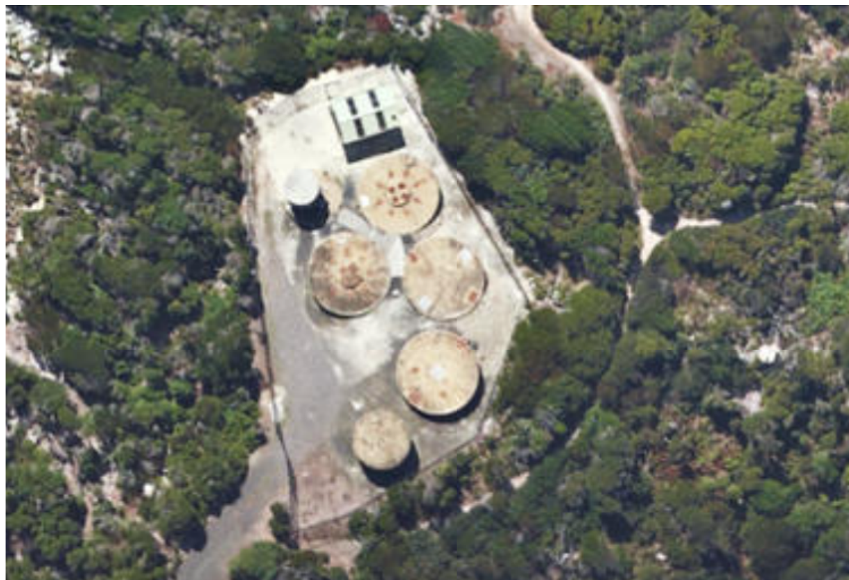
Figure 5-1: Boat Harbour Sewage Treatment plant
