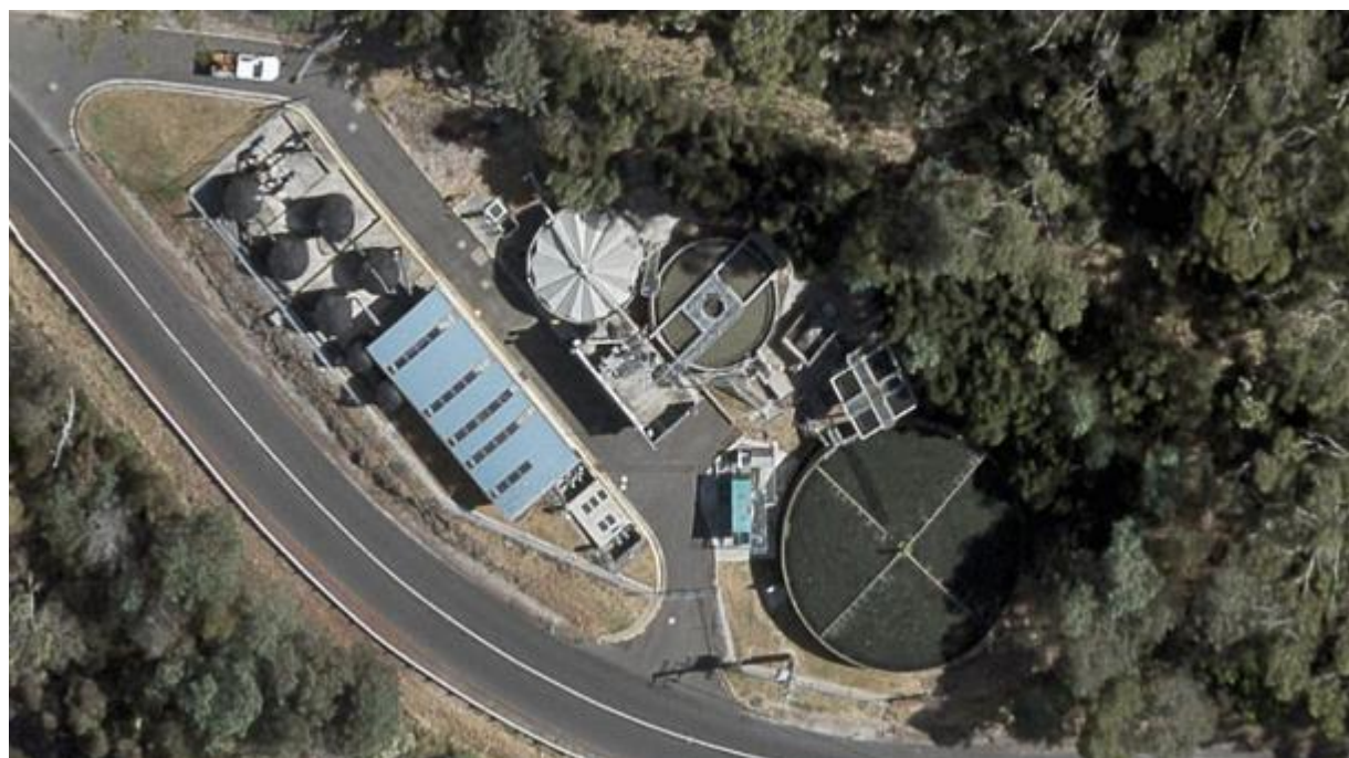
Figure 29-1: Latrobe Sewage Treatment Plant
