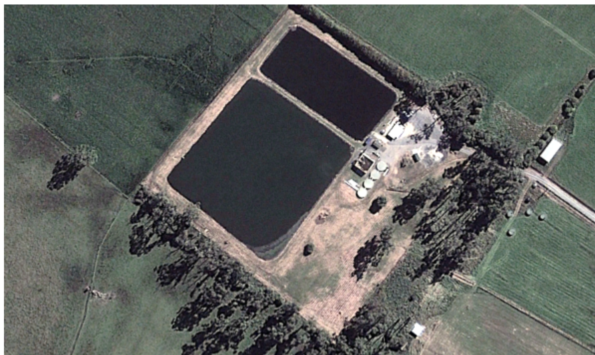
Figure 58-1: Sheffield Sewage Treatment Plant
