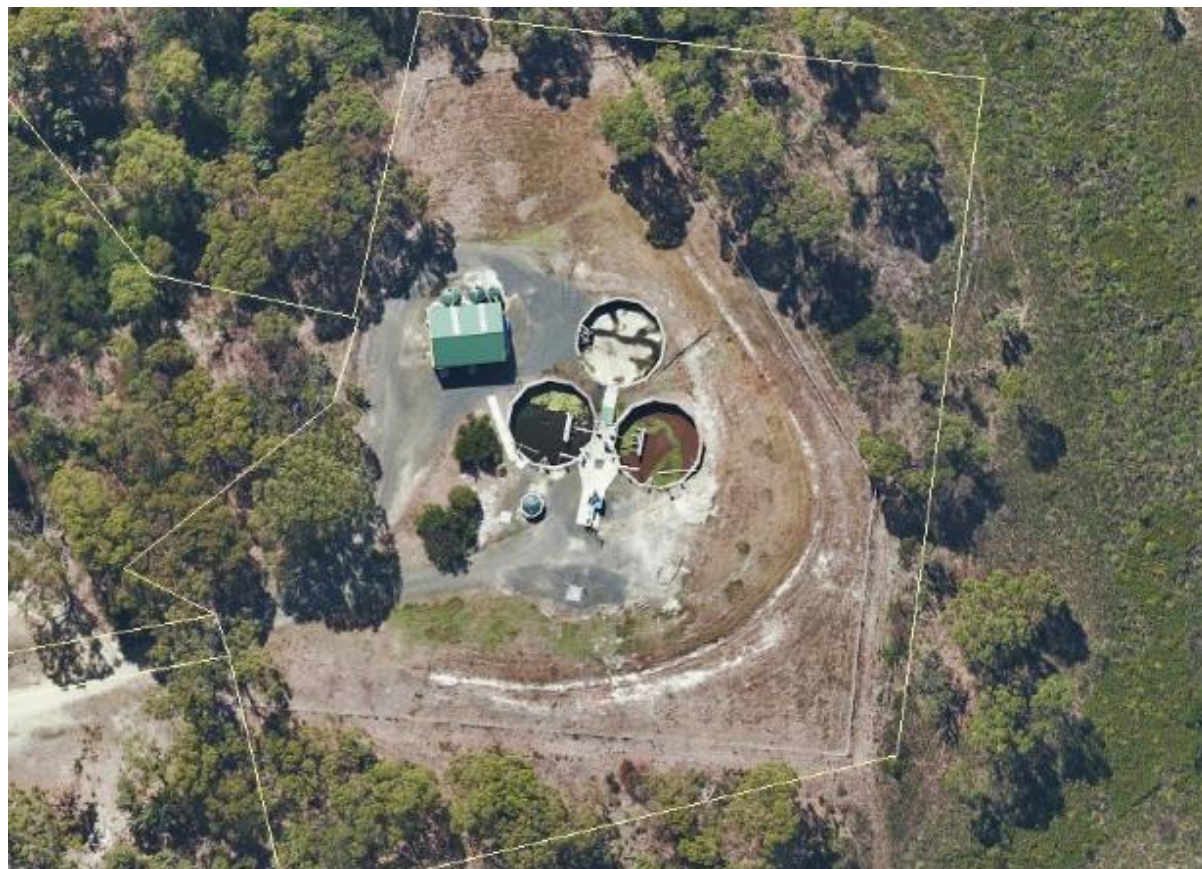
Figure 59-1: Sisters Beach Sewage Treatment Plant
