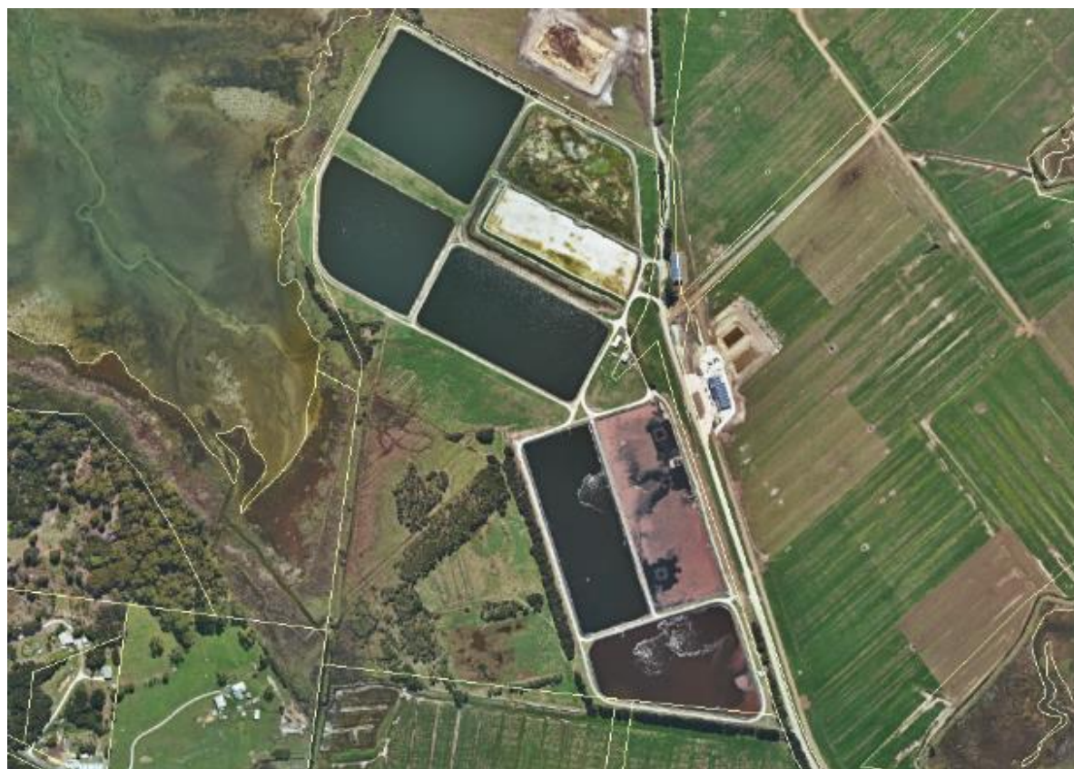
Figure 60-1: Smithton Sewage Treatment Plant
