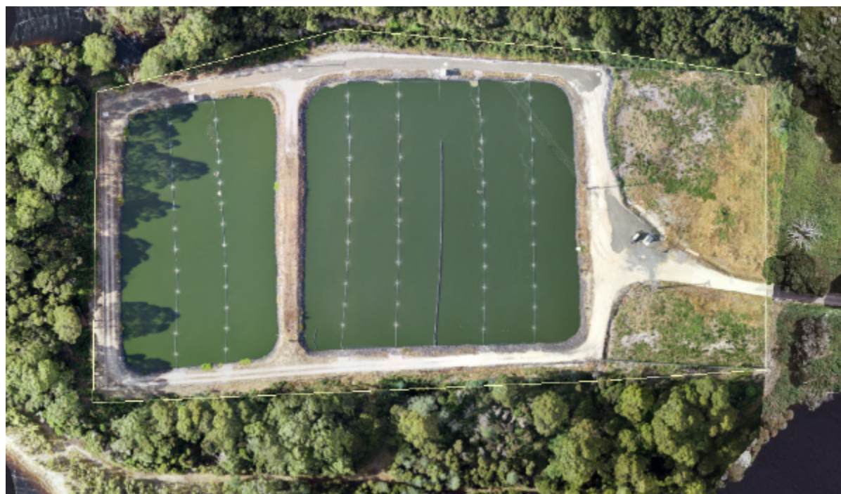
Figure 71-1: Tullah Sewage Treatment Plant
