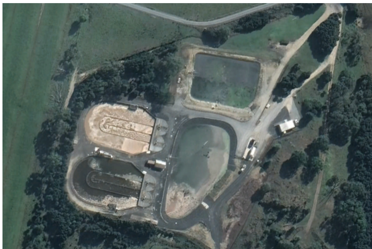
Figure 76-1: Wynyard Sewage Treatment Plant
