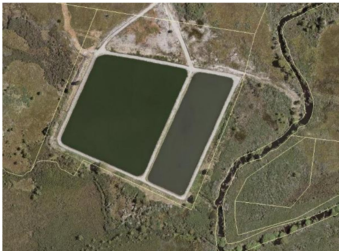
Figure 77-1: Zeehan Sewage Treatment Plant
