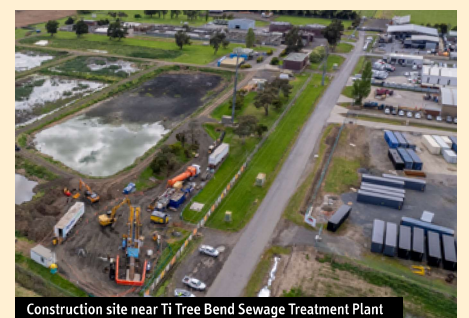
Construction site near Ti Tree Bend Sewage Treatment Plant
